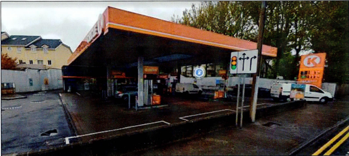
Figure 2 – View of Service Station (Source: Google Maps, 2022)
